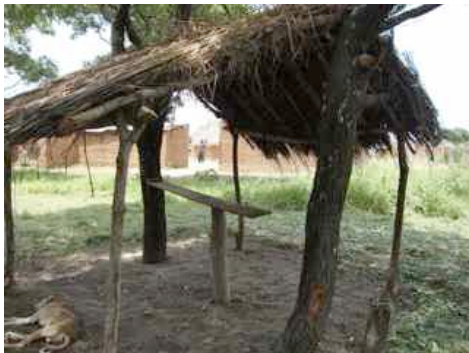
Shelter for the Carpenters made in Chimbalu Village
